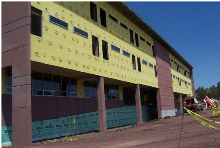
Figure 16 – Walkway during construction
