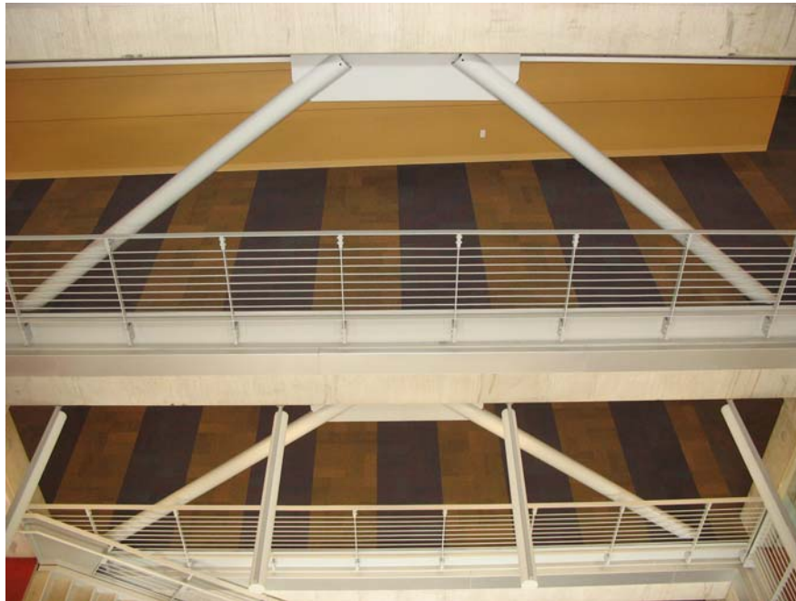
Figure 7 – Braced Frame in Completed CBA
