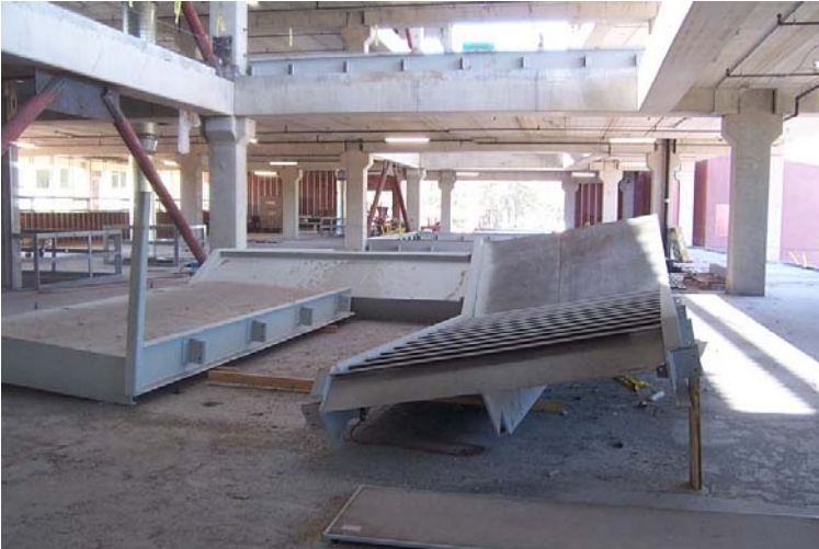
Figure 25 – CBA under construction
